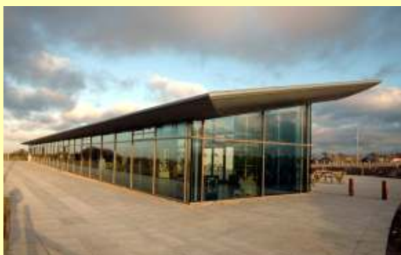
The new Chilterns Gateway Centre at Dunstable Downs
