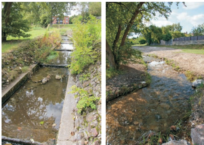
The R. Wye at Desborough Recreation Ground in High Wycombe, before and after restoration work.
