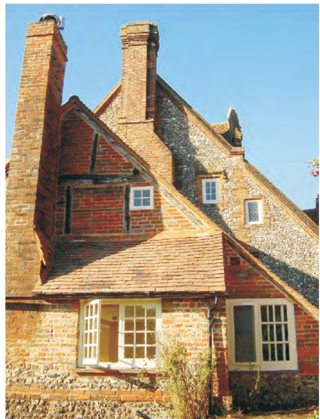
Sensitive extension to traditional building
